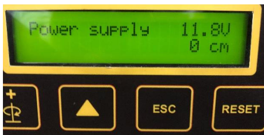
Current power supply and depth
